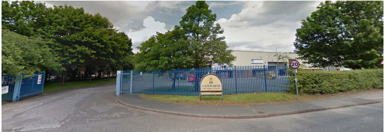
View of Units 1-11 Gatewarth Industrial Estate
